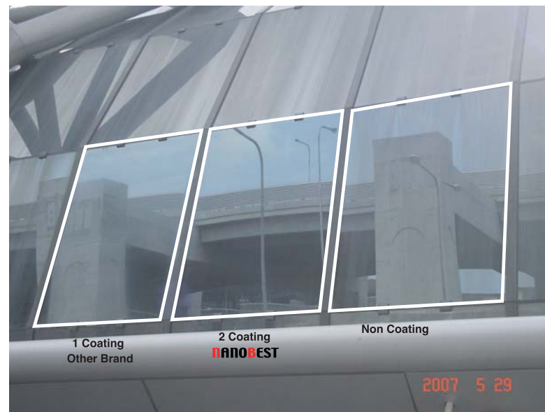
▲ 20 days after the coating clear difference compared to the other product applied on left
